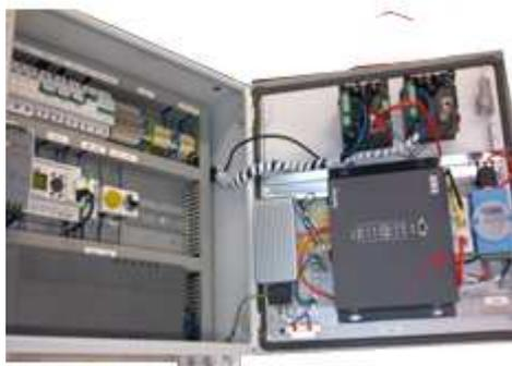
Figure 5: Cabinet with all system equipment
